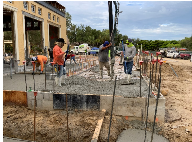
Pouring the foundation for expanded cardio area
