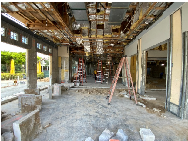
Concrete floor cutouts for new electrical floor boxes
