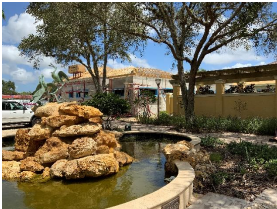
Trusses Installed over Group Fitness Room
