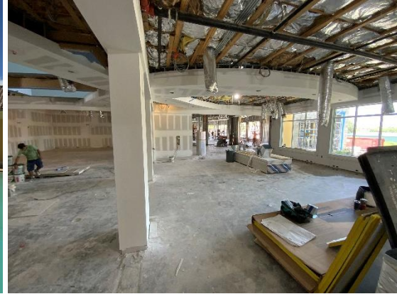
New Construction including Pool Entrance Installation of Drywall Walls/Soffit Ceiling
