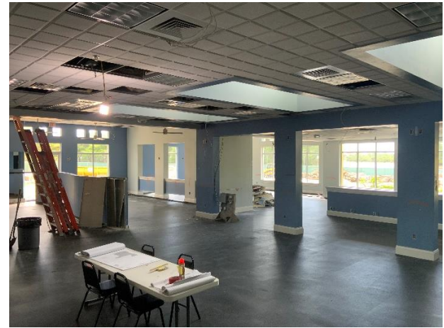
Interiors prepped for demoliton starting on Monday
