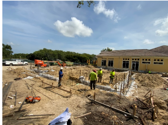
New west wall – adjacent to new group exercise space
