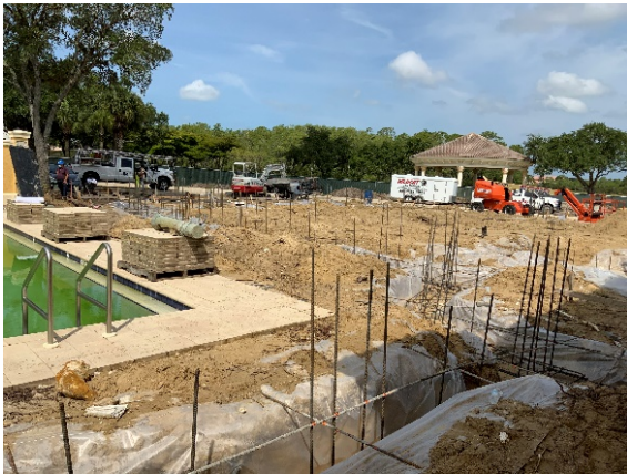
Construction of new pool entrance from interior
